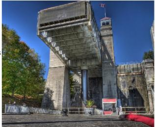
The tanks hold the same nominal amounts of water, so that the tanks are more or less balanced. This still applies when boats enter the tanks, because Archimedes Principle decrees that boats displace their own mass of water.
